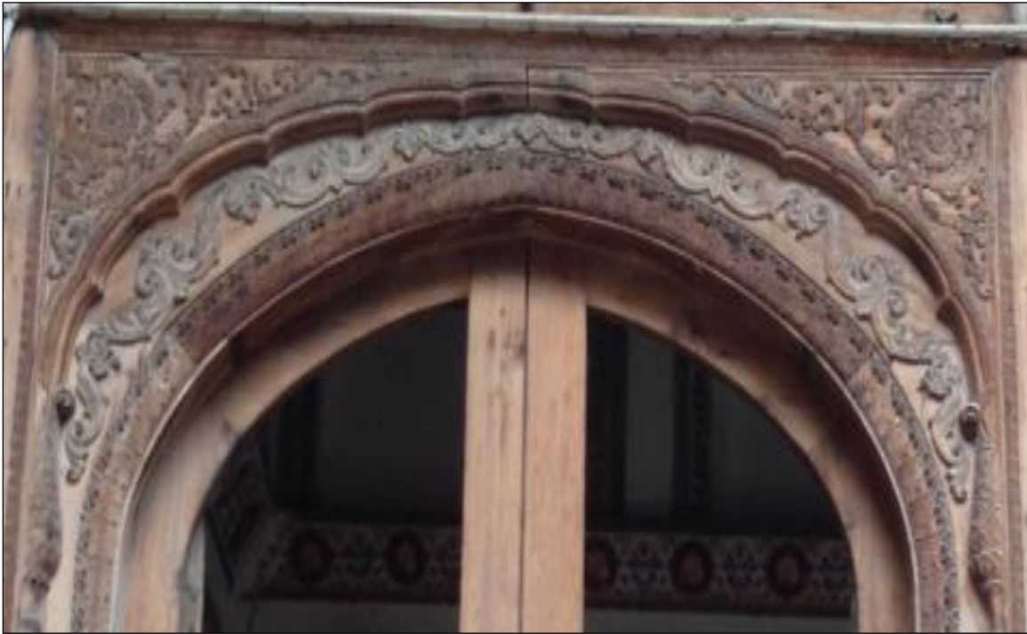
Figure.8. Rosettes on both sides of the spandrel floral scrolls spreading out towards both ends
