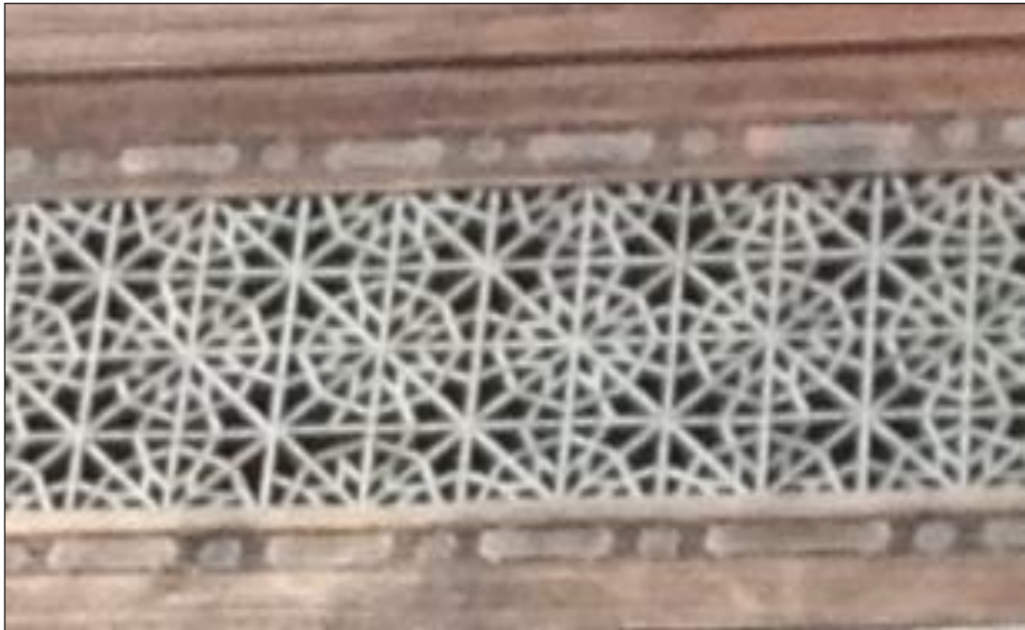
Figure.4. lattice work showing circle-shaped patterns containing stars in traditional building of Peshawar
